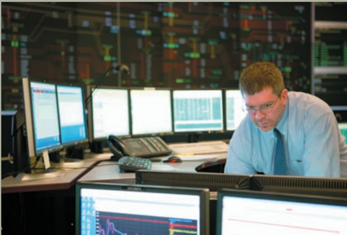
IESO Control Room
